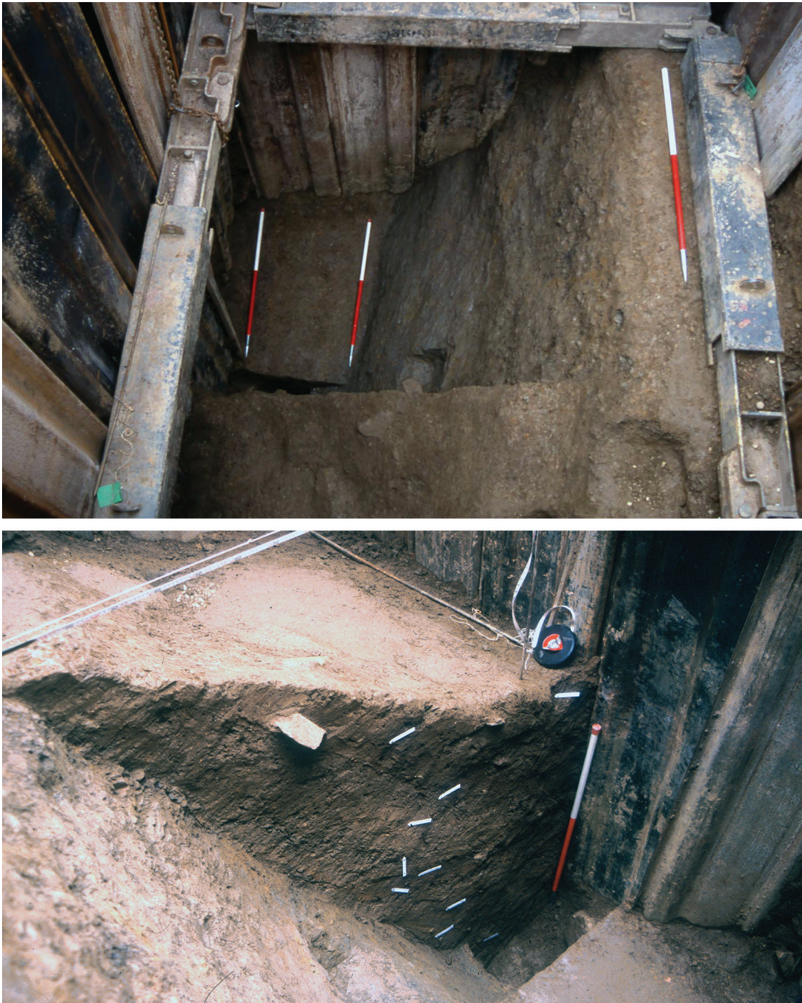
Figure 7.1: The east moat of the castle as exposed in the excavations conducted by ARCUS in 1999. These photographs show the metal shoring used in modern excavations, which is a great contrast with the ways in which the walls of trenches were braced in the early and middle decades of the 20th century, when timber, sometimes just reused doors, was used, if anything. University of Sheffield.
