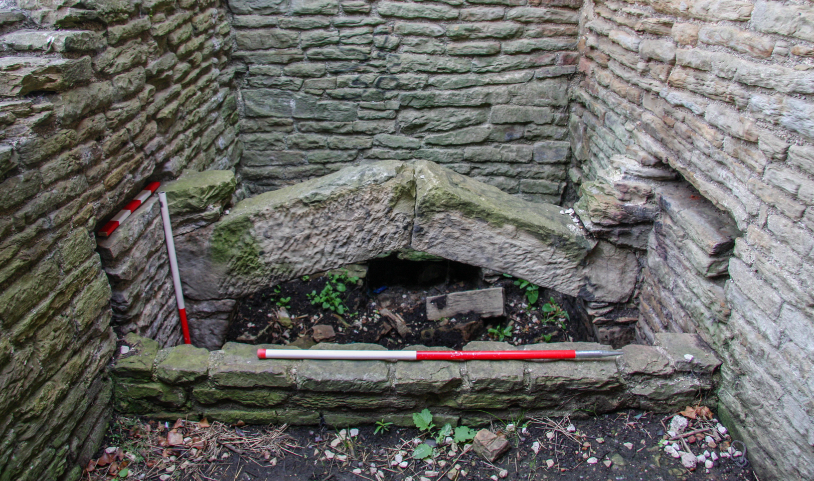
Figure 8.16: The garderobe in the three-storey tower. It takes the form of a low stone arch across the room; there was an associated timber structure and a drain leading through the north wall. Wessex Archaeology.
