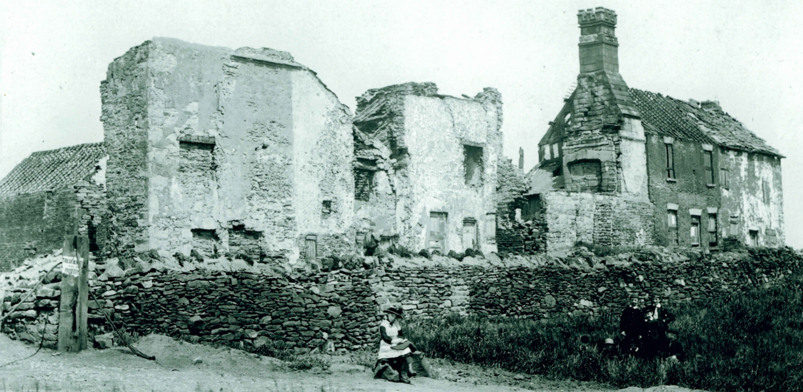
Figure 8.23: The south service range photographed in the late 19th century. It had once housed cottages for workers in the mining industry and the Norfolk Arms pub. The pub had been in the second cottage from the right; above the door are traces of its licencing information, and the hole visible higher up the wall was where the signage was formerly fixed. The roof next to the large tower had collapsed, and a first-floor fireplace is visible. The photograph has been annotated to suggest it was part of a series of postcards issued by a company called JWM and RPS; by now the former hunting lodge was becoming a local curiosity. Courtesy of Museums Sheffield.
