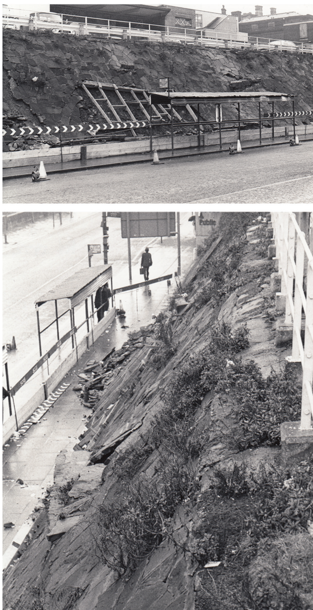
Figure 1.16: Collapse of the retaining wall above Castlegate in 1972. A section of castle wall is visible above the right-hand end of the bus stop (top) and another at the lower part of the slope (below). Recording of these exposed parts of the castle was undertaken by Pauline Beswick of Sheffield City Museum. Courtesy of Museums Sheffield.
