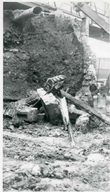
47 Filling behind B & C ret. wall appears to have carried away upper part of slope of moat seen in T.H.C (see 17)
