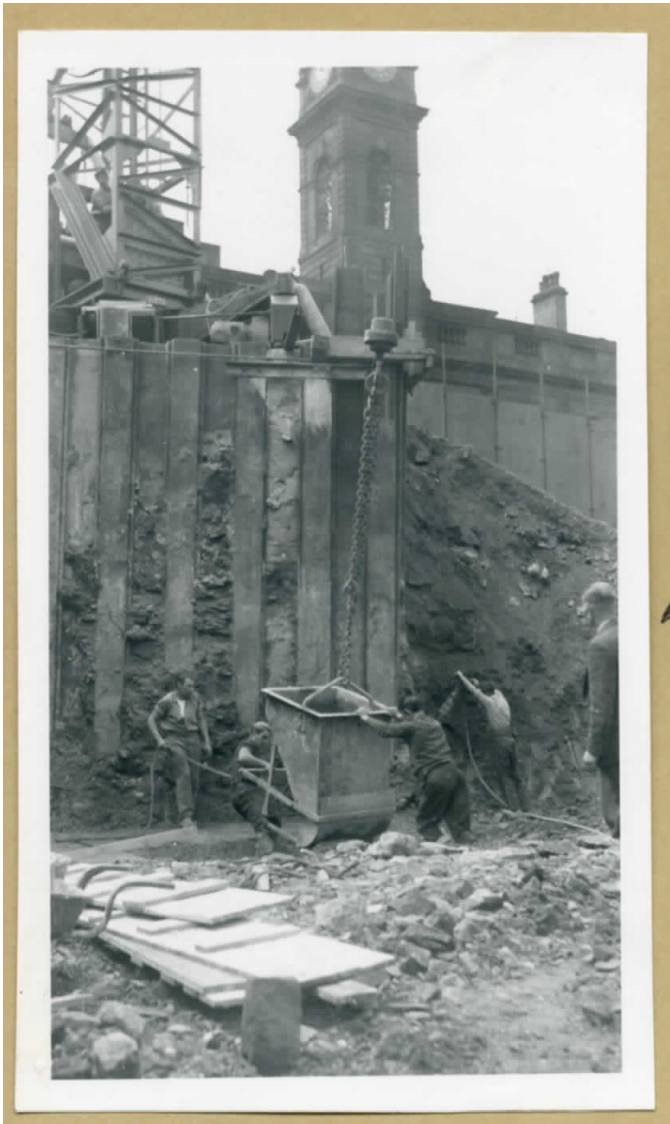
Figure 4.8: Workmen filling a bucket – or kibble as it was known in mining parlance – during construction work on Exchange Street. Courtesy of Museums Sheffield.
