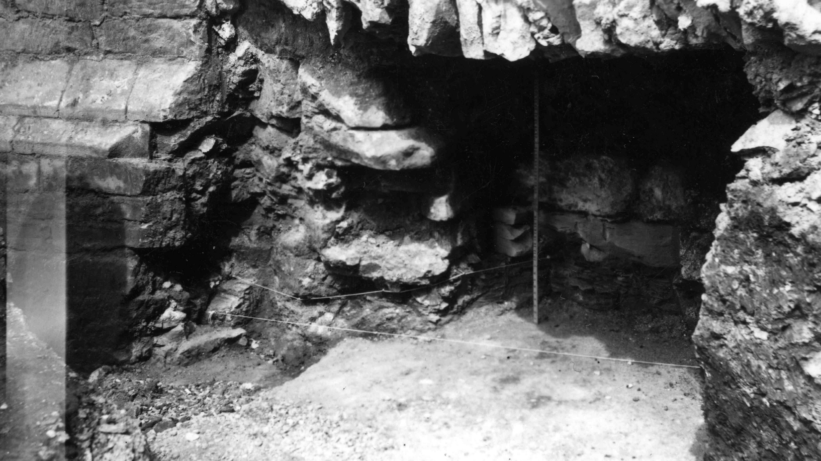
Figure 4.18: Photograph taken near the gatehouse showing how the foundation shafts were strung up for recording. Courtesy of Museums Sheffield.
