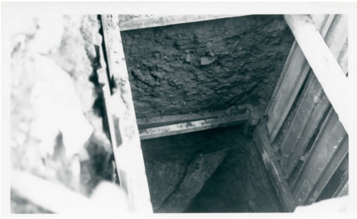
Figure 5.3: Looking down foundation shaft E19 from the north-east. This photograph shows the use of shuttering by the construction workers. Courtesy of Museums Sheffield.
